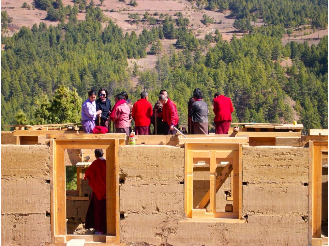
Nuns building their own monastery in a traditional, pounded-earth technique. Some people believe that traditional structures are stronger during earthquakes than concrete buildings. 尼師門運用傳統的夯土方式建造她們的寺院。一些人認為傳統結構在地震中比水泥更結實。
