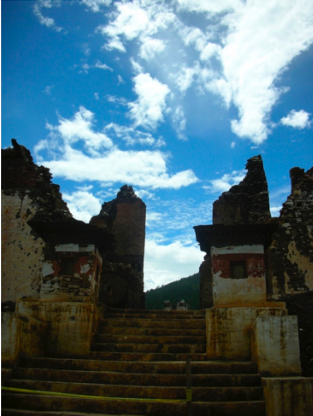
Entire historic monastery burned down due to electrical fire
